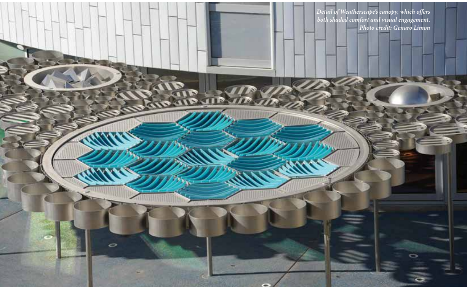
The exterior and interior skins of the structure are geometrically similar, but materially distinct tessellated and shingled modules. The highly reflective exterior is contrasted by a tactile and colourful interior. Photo credit: Matthew Millman
